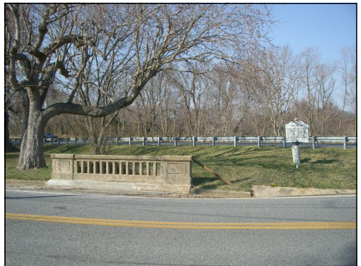
At Linchester Mills, an example of early roadway feature that should be preserved.
