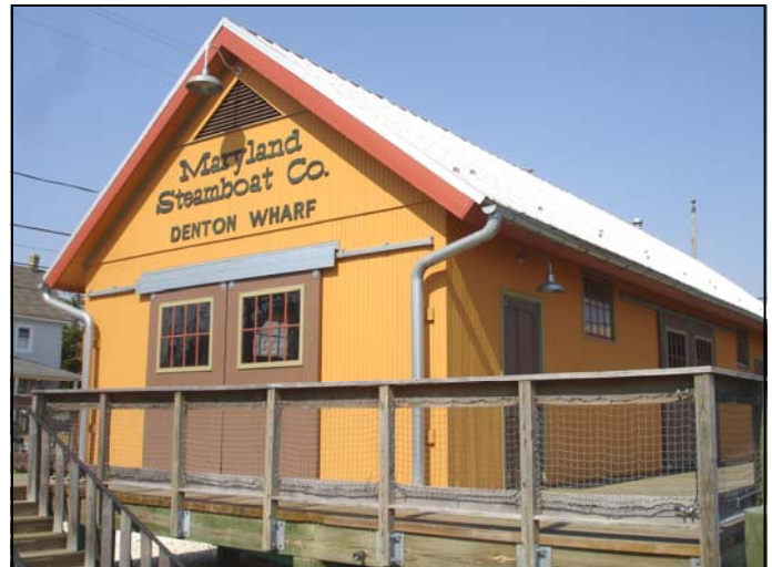
The wharf at Denton has been restored.
